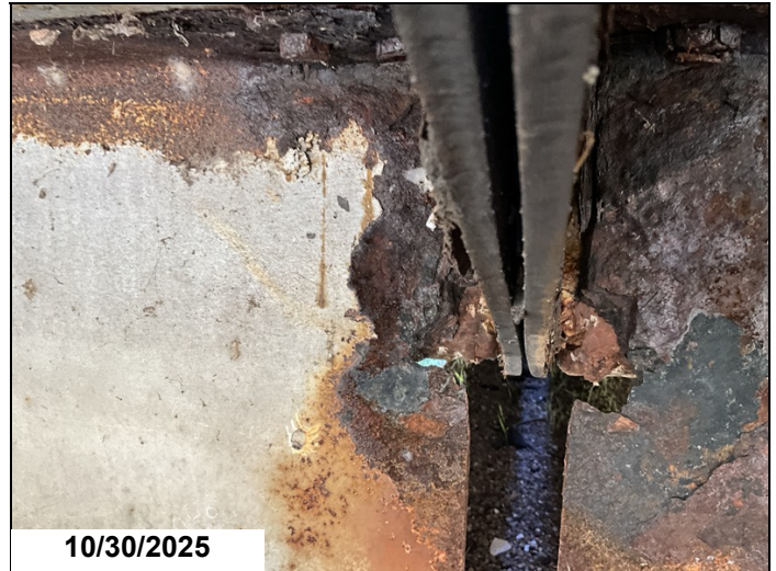
Span 14 bent 14 girder 1 has a 2" x 3" hole in web below haunch 1LF CS3.
