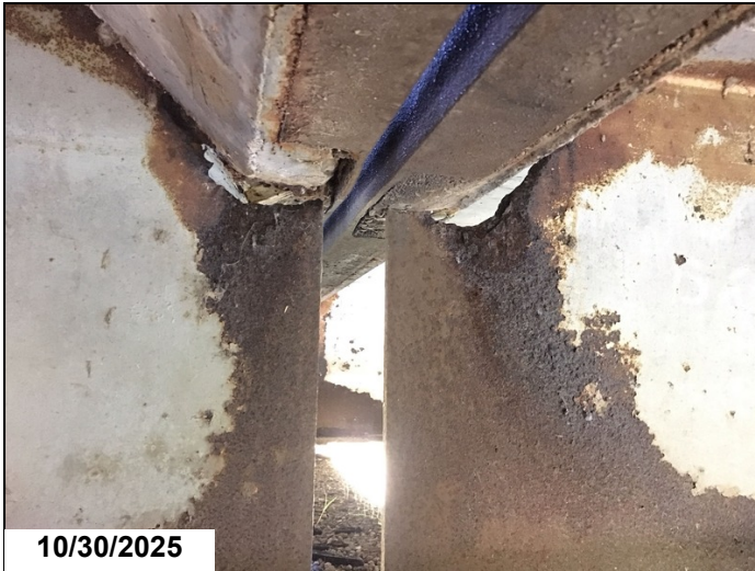
Span 13 bent 14 girder 2 has a 7" x 1" hole in web below haunch 1LF CS3.
