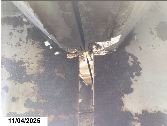
Span 19 bent 19 girder 2 has a 4.5" x 1" hole in web below haunch 1LF CS3.
