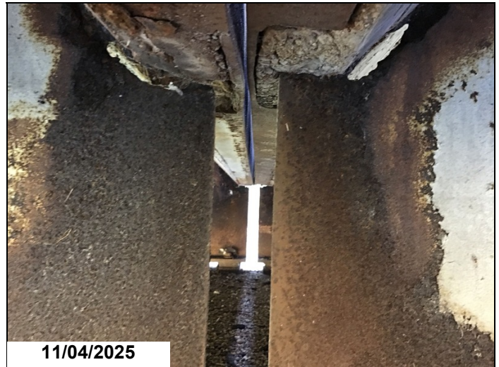
Span 15 bent 15 girder 3 has a 6" x 1" hole in web below haunch 1LF CS3.
