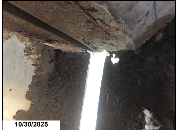
Span 13 bent 14 girder 4 has a 2" x 2" hole in web below haunch 1LF CS3.
