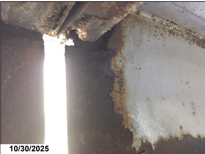
Span 9 bent 9 girder 1 has 1" diameter hole in web below haunch 1LF CS3.
