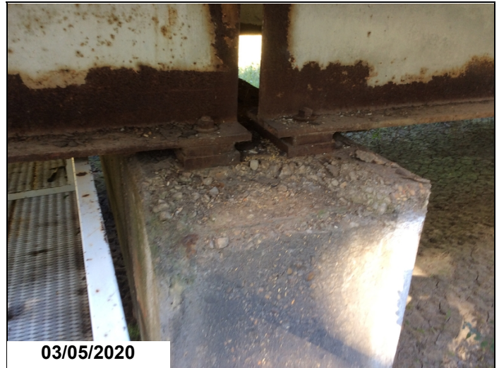
Bent 15 right end of cap under girder 4 bearings.
