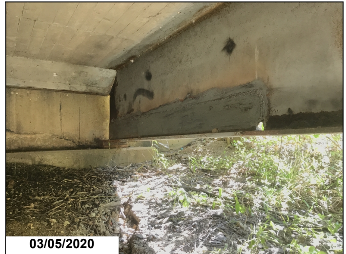
Span 21 bent 22 girder 4 bottom of web was t-spliced in the past, web below haunch has a 1" diameter hole 1LF CS3.
