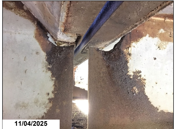
Span 14 bent 14 girder 2 has a 7" x 1.5" hole in web below haunch and girder is floating 1/16" 1LF CS3.
