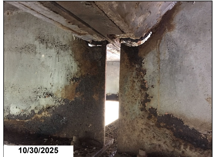
Span 1 bent 2 girder 2 has a 5" x 1" hole in web below haunch 1LF CS3.
