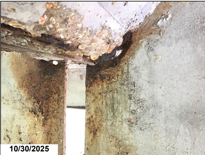
Span 2 bent 2 girder 3 has a 6" x 1" hole in web below haunch 1LF CS3.
