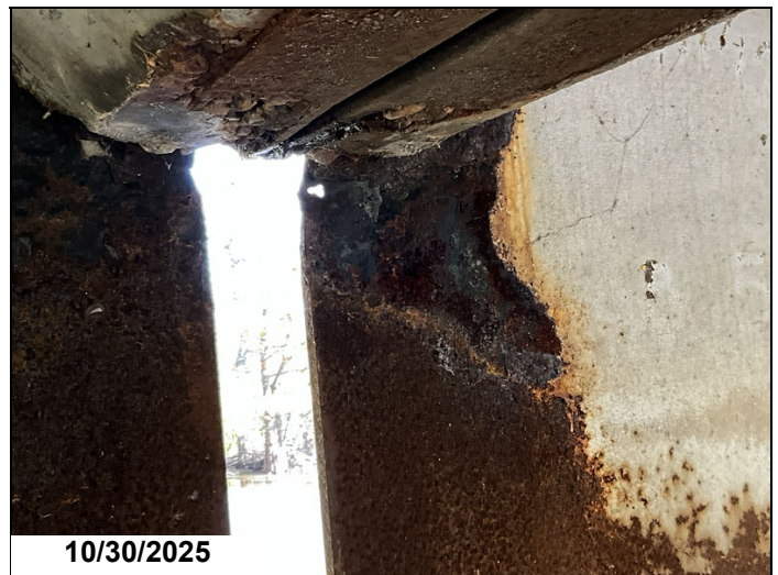
Span 20 bent 20 girder 1 has a 1" diameter hole in web below haunch 1LF CS3.
