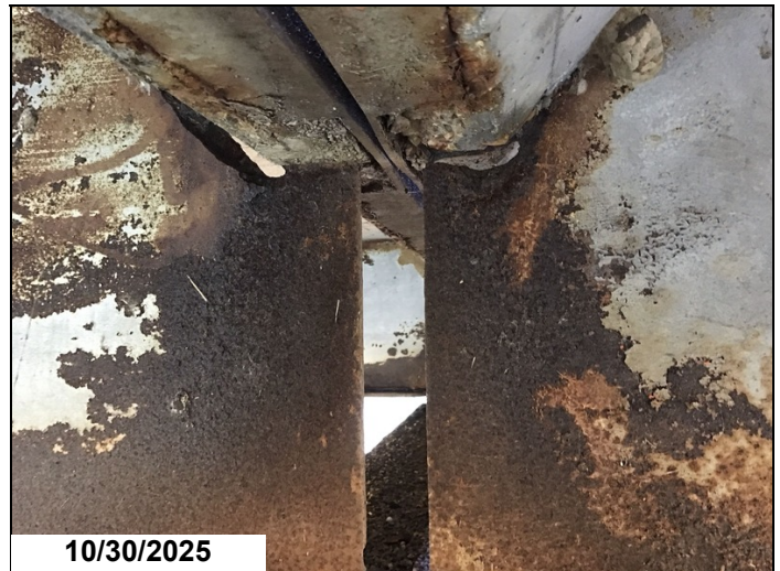
Span 6 bent 7 girder 2 has a 5" x 1" hole in web below haunch 1LF CS3.
