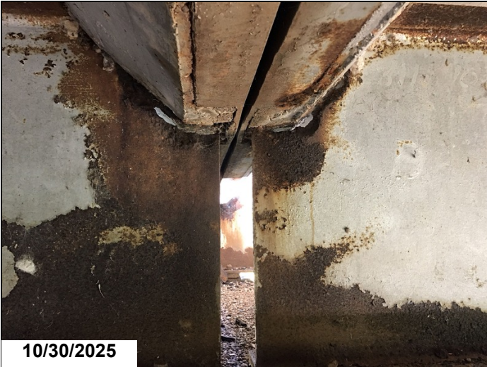
Span 15 bent 16 girder 2 has a 7" x 1" hole in web below haunch 1LF CS3.
