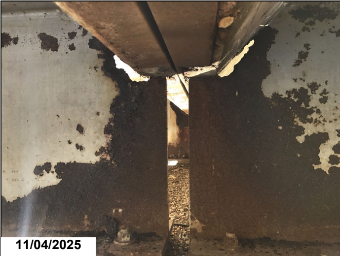
Span 20 bent 20 girder 3 has a 6" x 1" hole in web below haunch, with 2" crack running back 1LF CS3.
