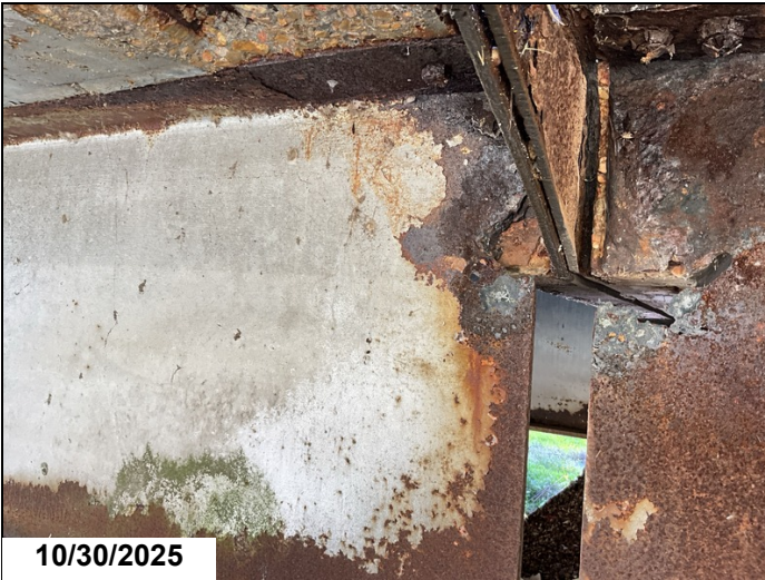
Span 17 bent 17 girder 1 has a 6" x 4" area in web below haunch, with holes rusted through 1LF CS3.
