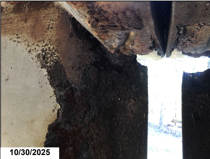
Span 16 bent 16 girder 4 has a 2" diameter hole in web below haunch 1LF CS3.
