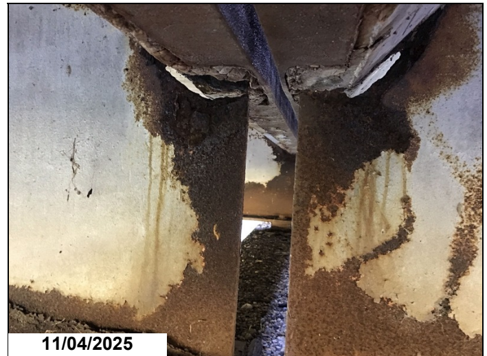
Span 12 bent 12 girder 3 has a 7" x 1" hole in web below haunch 1LF CS3.
