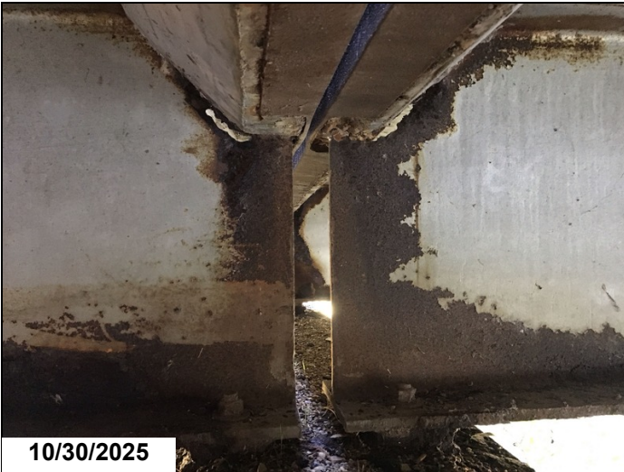
Span 10 bent 11 girder 2 has a 4" x 1" hole in web below haunch 1LF CS3.
