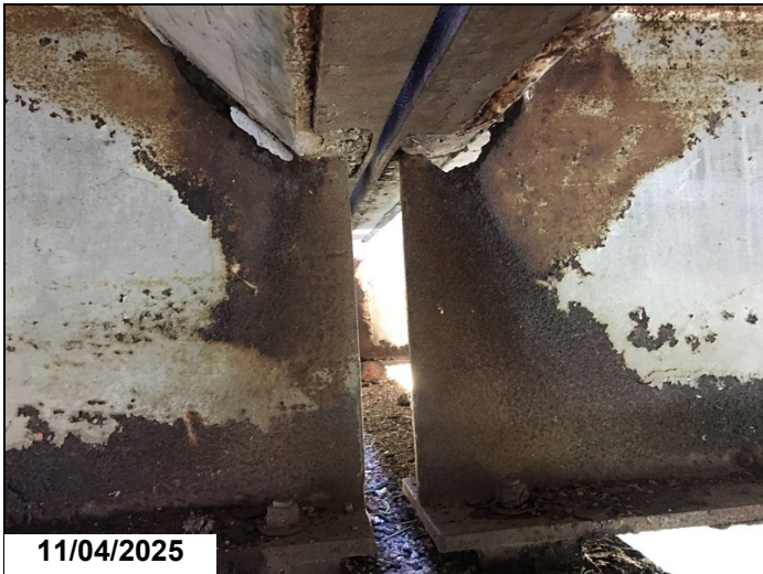
Span 15 bent 15 girder 2 has a 5" x 1" hole in web below haunch, with a 2" crack running ahead 1LF CS3.
