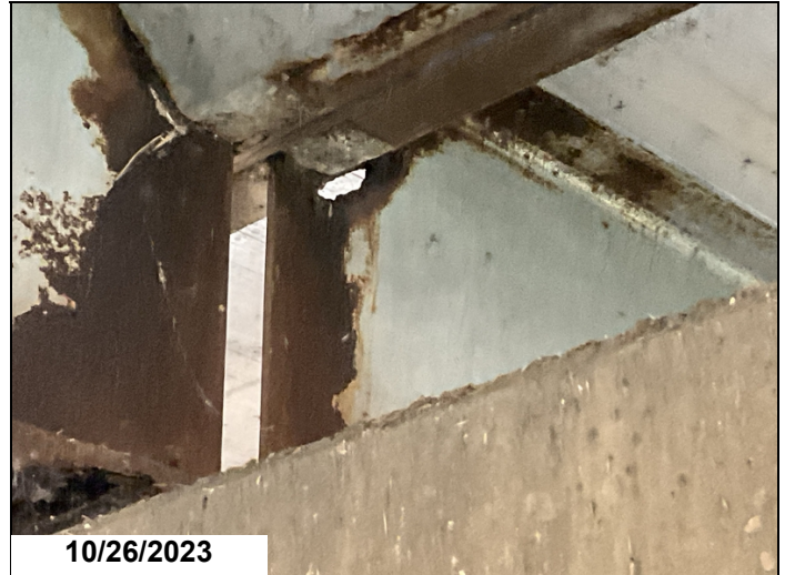
Span 6 bent 7 girder 3 has a 6" x 1" hole in web below haunch 1LF CS3.
