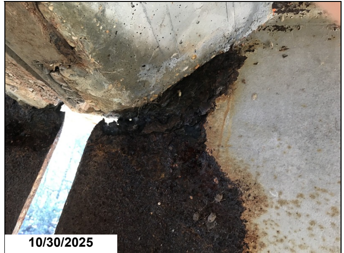
Span 18 bent 19 girder 4 has a 3" x 1" hole in web below haunch 1LF CS3.
