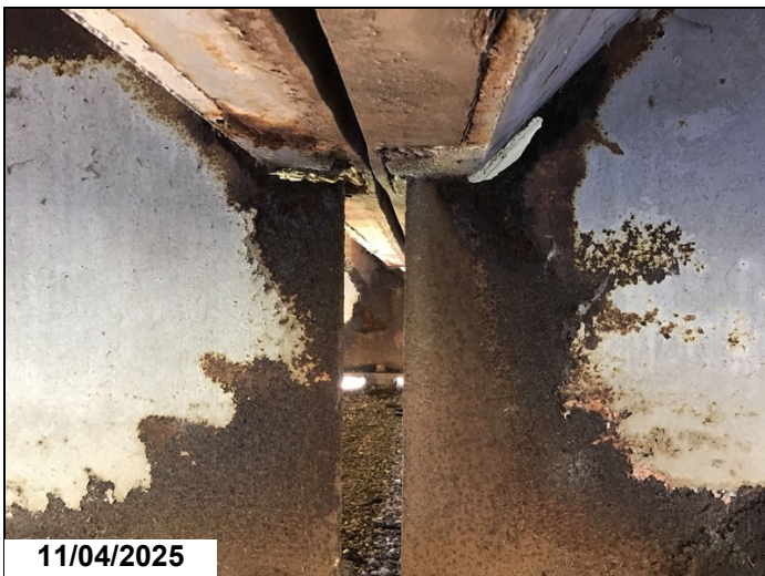
Span 16 bent 16 girder 3 has a 4" x 1" hole in web below haunch 1LF CS3.
