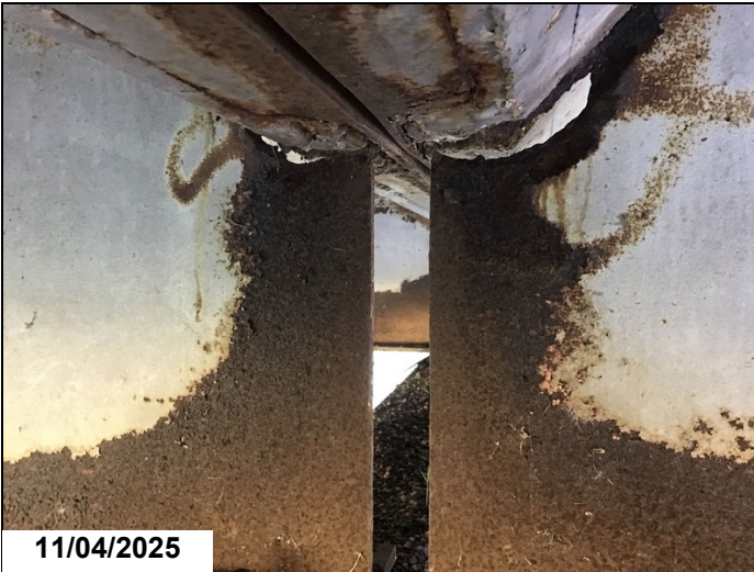
Span 9 bent 9 girder 3 has a 6" x 1" hole in web below haunch 1LF CS3.
