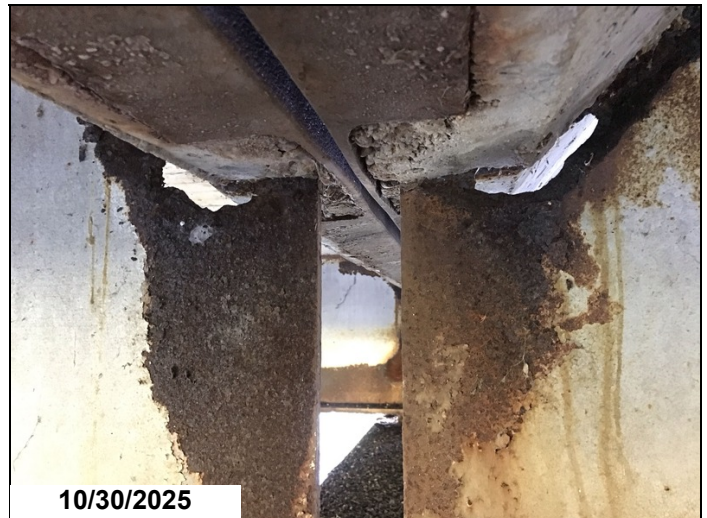
Span 10 bent 11 girder 3 has a 5" x 1" hole in web below haunch 1LF CS3.
