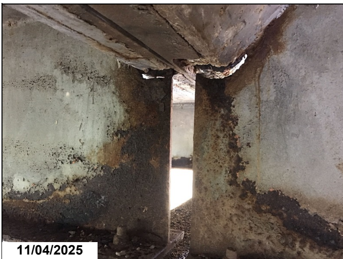
Span 2 bent 2 girder 2 has a 6" x 1" hole in web below haunch 1LF CS3.
