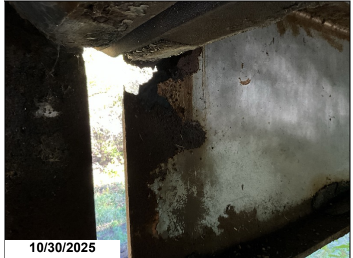
Span 13 bent 13 girder 1 has a 4" x 3" hole in web below haunch 1LF CS3.
