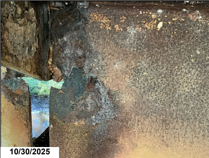
Span 13 bent 14 girder 1 has a 2" x 3" hole in web below haunch 1LF CS3.
