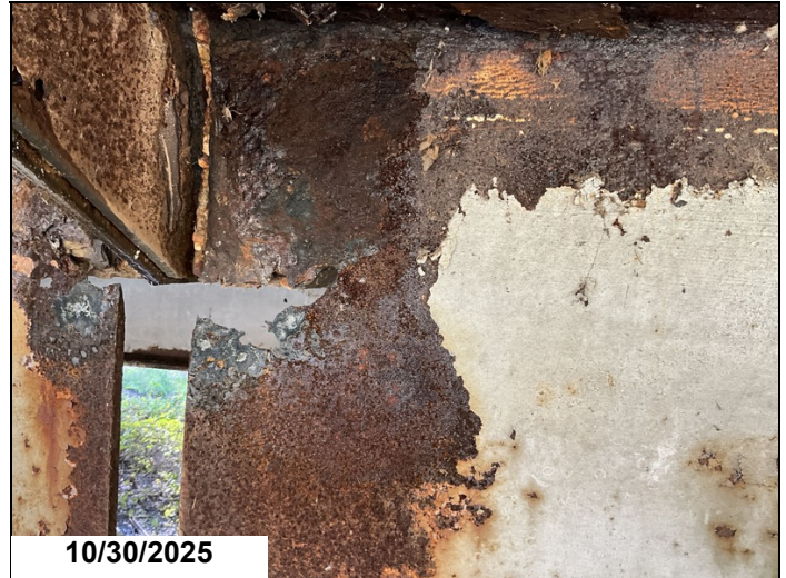
Span 16 bent 17 girder 1 has a 6" x 3" hole in web below haunch, with a 1" crack running back 1LF CS3.
