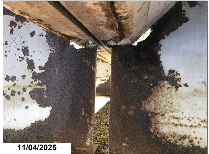
Span 19 bent 19 girder 3 has a 9" x 1" hole in web below haunch, with a 1" crack running back 1LF CS3.
