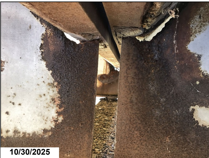
Span 17 bent 18 girder 3 has a 7" x 1" hole in web below haunch, with a 2" crack running ahead 1LF CS3.
