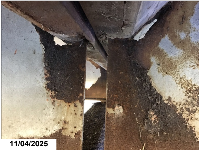
Span 13 bent 13 girder 3 has a 5" x 1" hole in web below haunch 1LF CS3.
