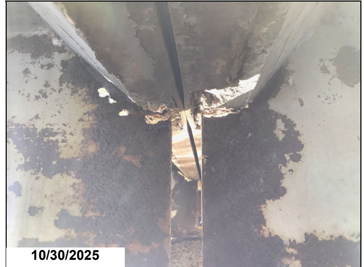
10/30/2025 Span 18 bent 19 girder 2 has a 5" x up to 1" hole in web below haunch 1LF CS3.
