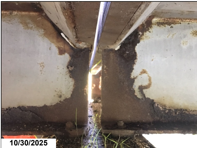
Span 11 bent 12 girder 2 has a 10" x 1" hole in web below haunch 1LF CS3.
