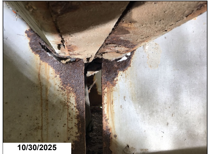
Span 19 bent 20 girder 2 has a 6" x 1" hole in web below haunch, with a 1" crack running ahead 1LF CS3.
