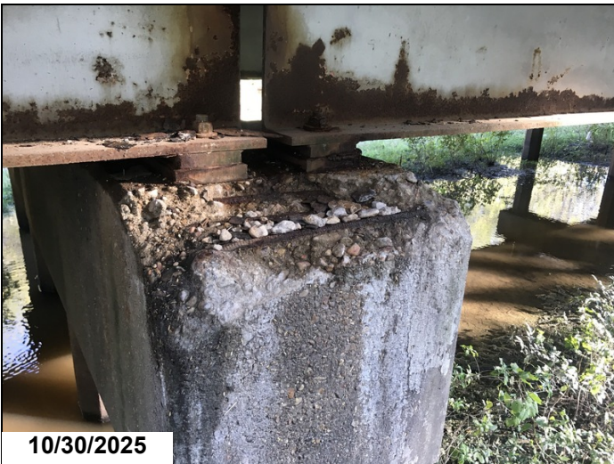
Bent 14 cap right end has a 1' spall near bearing area with exposed rebar CS3.
