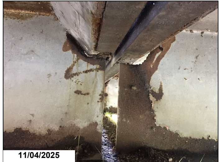
Span 13 bent 13 girder 2 has a 6" x 2" hole in web below haunch 1LF CS3.
