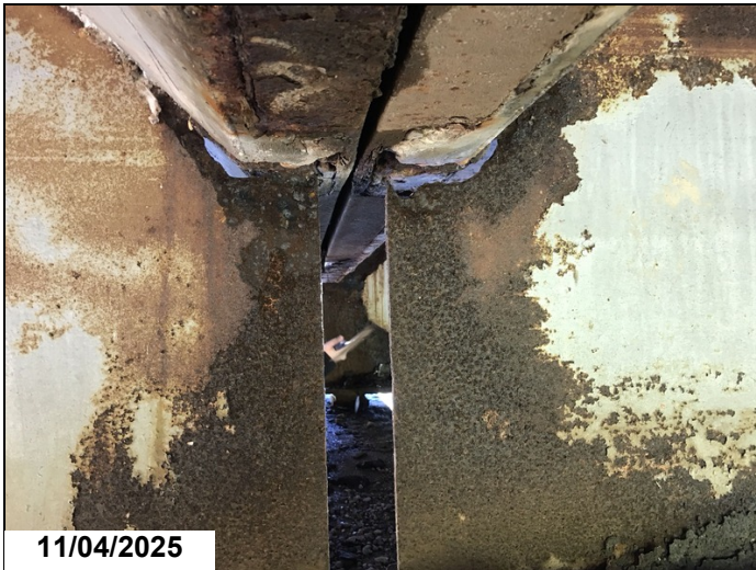
Span 21 bent 21 girder 2 has a 6" x 1" hole in web below haunch 1LF CS3.
