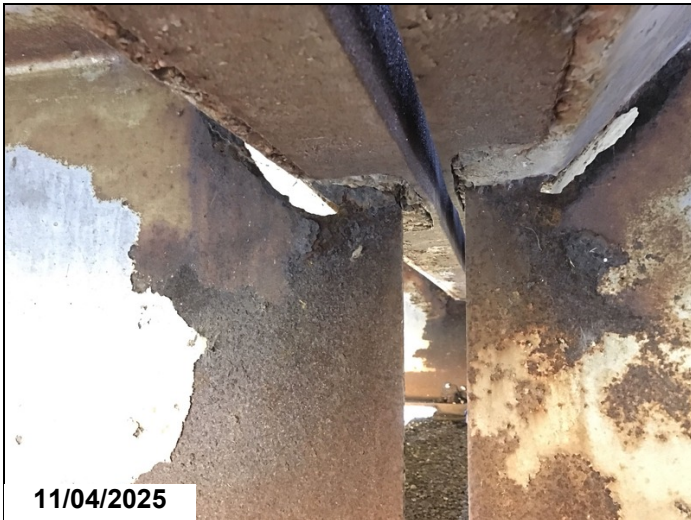
Span 14 bent 14 girder 3 has a 7" x 1" hole in web below haunch 1LF CS3.
