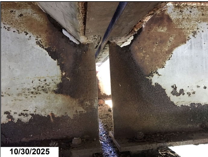
Span 14 bent 15 girder 2 has a 5" x 1" hole in web below haunch 1LF CS3.
