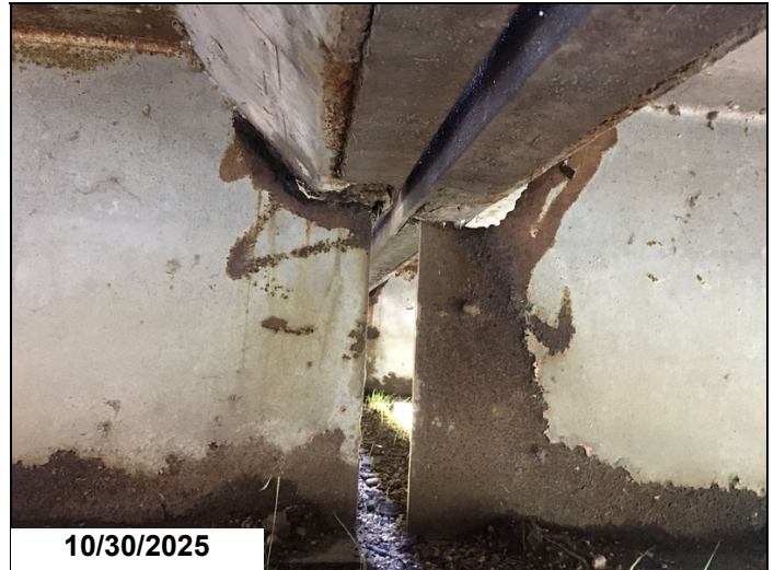
Span 12 bent 13 girder 2 has a 6" x 1" hole in web below haunch 1LF CS3.
