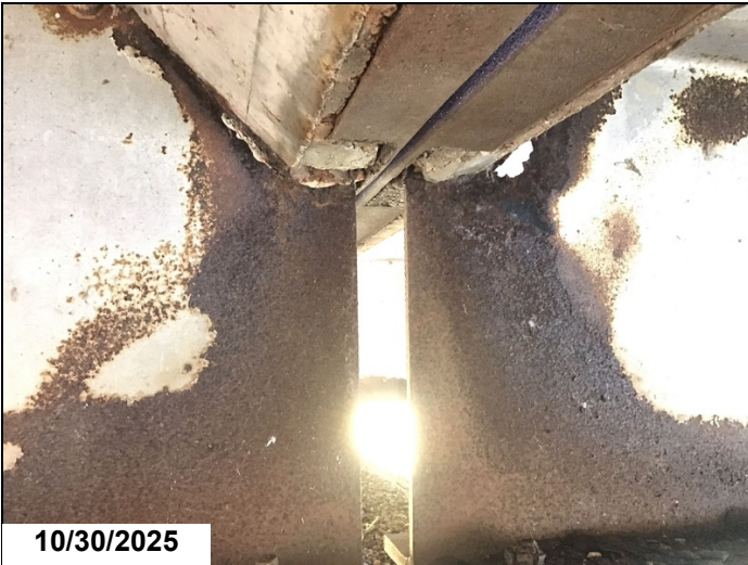
Span 9 bent 10 girder 2 has a 9" x 1" hole in web below haunch, with a 1" crack running ahead 1LF CS3.
