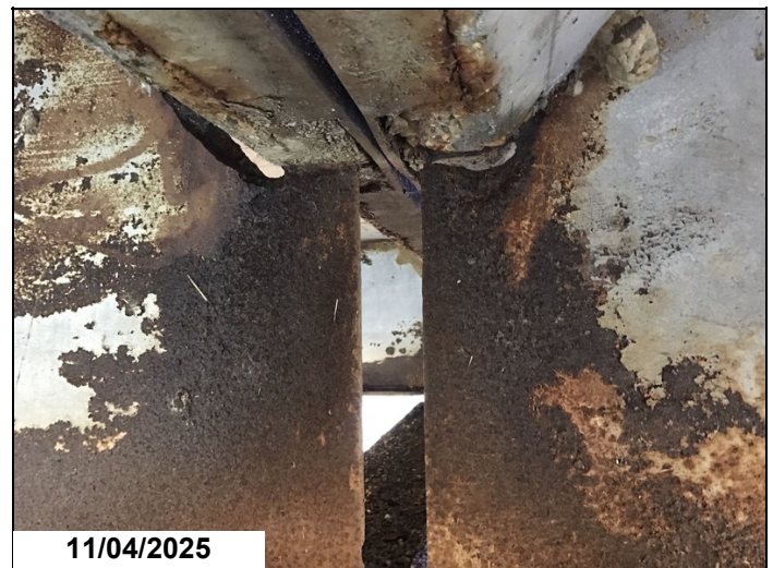
Span 7 bent 7 girder 2 has a 5" x 1" hole in web at haunch 1LF CS3.
