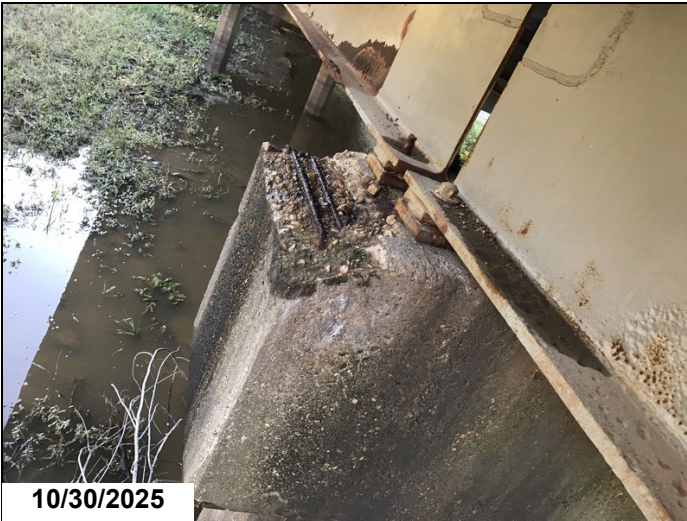
Bent 3 left has a 1' spall with exposed rebar. rebar CS3.
