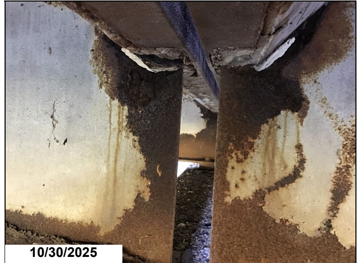
Span 11 bent 12 girder 3 has 5" x 1" hole in web below haunch 1LF CS3.
