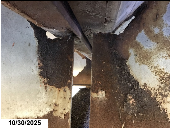
Span 12 bent 13 girder 3 has a 5" x 1" hole in web below haunch 1LF CS3.
