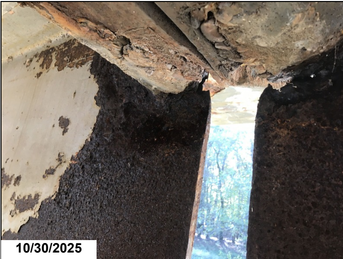
Span 19 bent 19 has a 1" hole in web below haunch.
