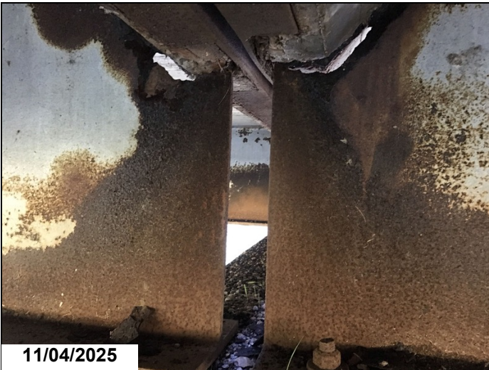
Span 10 bent 10 girder 3 has a 5" x 1" hole in web below haunch 1LF CS3.
