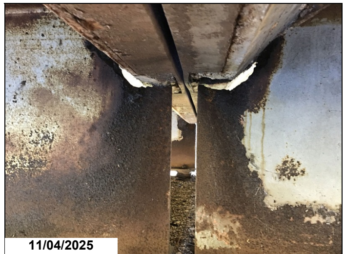
Span 17 bent 17 girder 3 has a 5" x 1" hole in web below haunch 1LF CS3.
