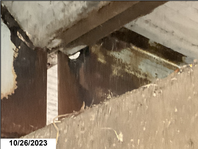
Span 7 bent 8 girder 3 has a 5" x 2" hole in web below haunch 1LF CS3.
