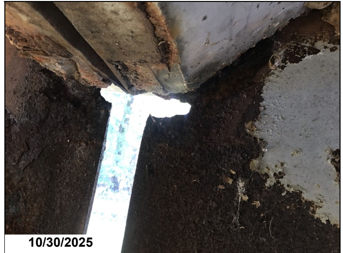
Span 15 bent 16 girder 4 has a 3" x 1" hole in web below haunch.
