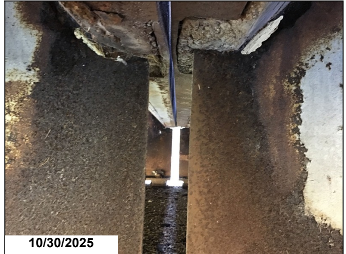
Span 14 bent 15 girder 3 has a 4" x 1" hole in web below haunch 1LF CS3.
