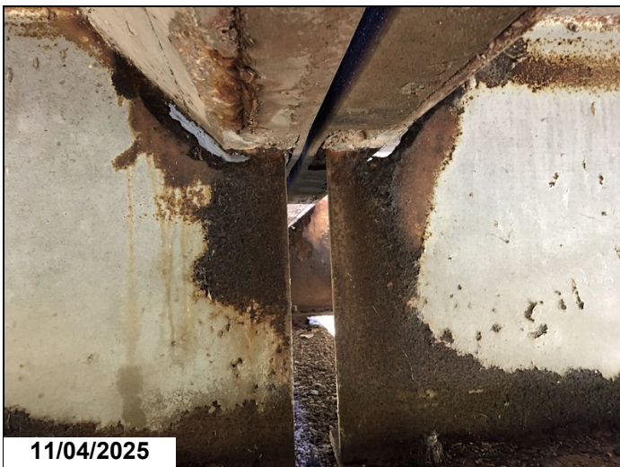
Span 17 bent 17 girder 2 has a 5" x 1" hole in web below haunch, with a 2" crack running ahead 1LF CS3.
