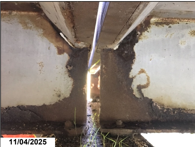
Span 12 bent 12 girder 2 has a 3" x 1" hole in web below haunch 1LF CS3.
