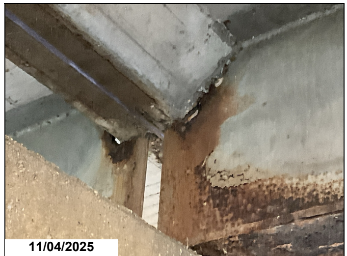
Span 6 bent 6 girder 3 has a 3" x 1" hole in web below haunch 1LF CS3.
