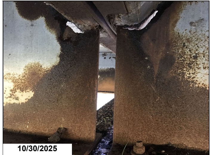
Span 9 bent 10 girder 3 has a 7" x 1" hole in web below haunch 1LF CS3.
