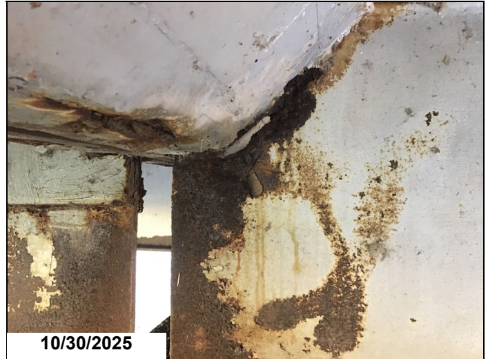
Span 8 bent 9 girder 2 has 3" x 1" hole in web below haunch 1LF CS3.
