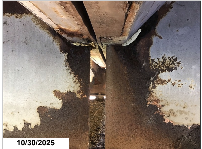
Span 15 bent 16 girder 3 has a 5" x 1" hole in web below haunch 1LF CS3.
