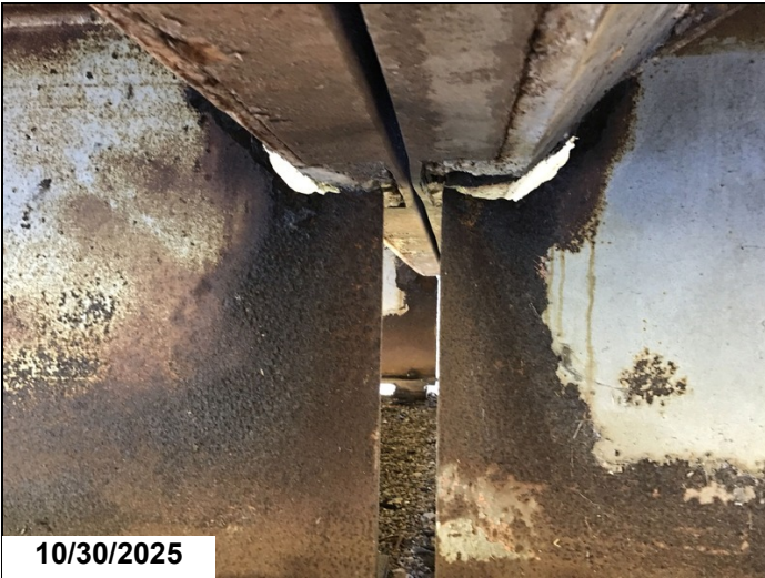
Span 16 bent 17 girder 3 has a 8" x 1" hole in web below haunch 1LF CS3.
