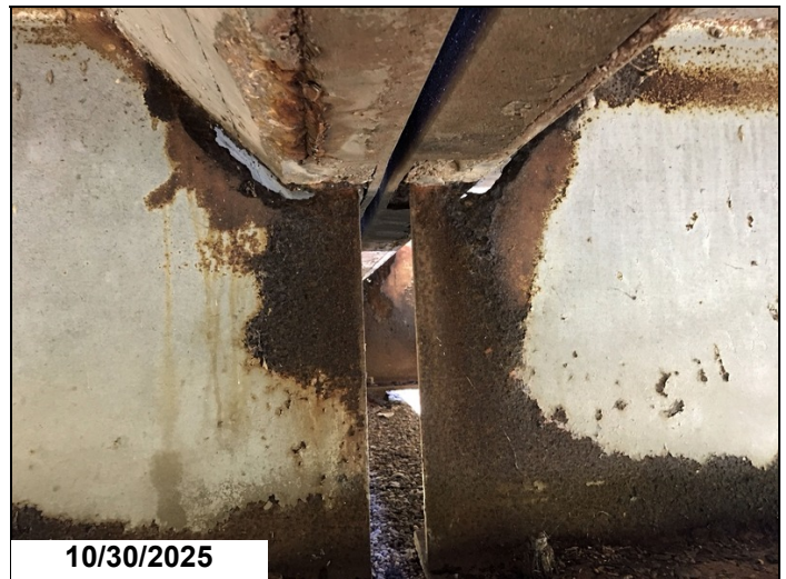
Span 16 bent 17 girder 2 has a 7" x 1" hole in web below haunch, with a 2" crack running ahead 1LF CS3.
