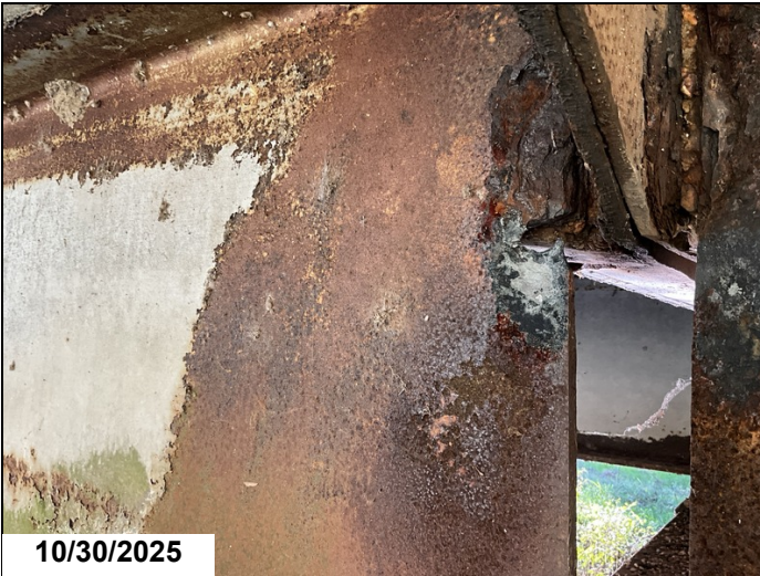
Span 16 bent 16 girder 1 has a 1" diameter hole in web below haunch, with a 1/4" crack running down and a 1/4" crack running ahead 1LF CS3.
