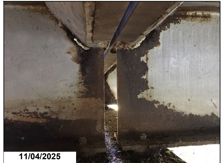
Span 11 bent 11 girder 2 has an 8" x 1" hole in web below haunch 1LF CS3.
