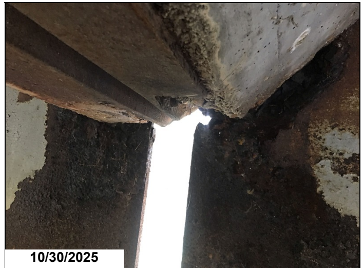
Span 12 bent 13 girder 4 has a 1" diameter hole in web below haunch 1LF CS3.
