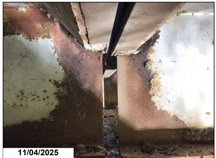
Span 18 bent 18 girder 2 has a 6" x 1" hole in web below haunch, with a 2" crack running back 1LF CS3.
