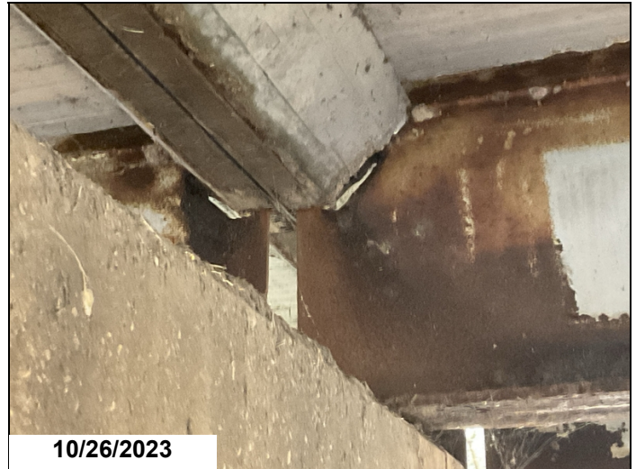
Span 7 bent 8 girder 2 has a 6" x 1" hole in web below haunch, with a 2" crack running ahead 1LF CS3.
