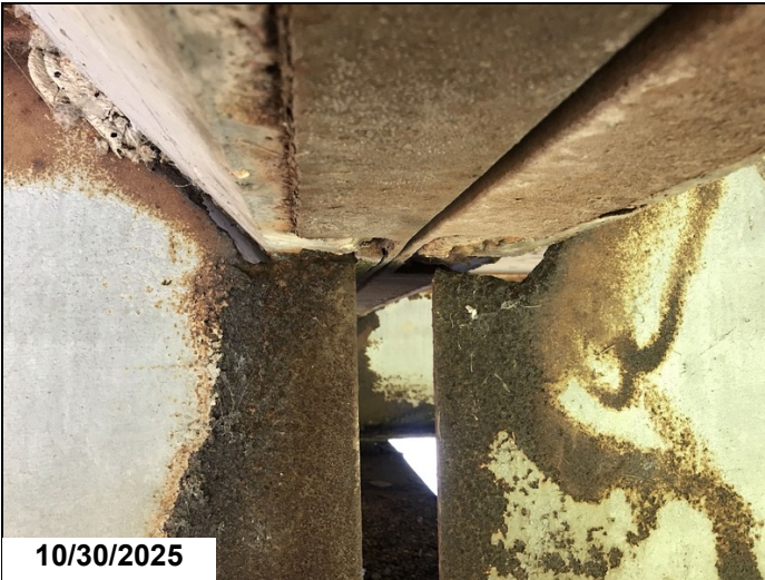
10/30/2025 Span 20 bent 21 girder 3 has a 4" x 1" hole in web below haunch, with a 2" crack running ahead 1LF CS3.
