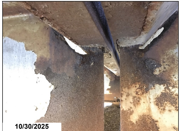
Span 13 bent 14 girder 3 has a 6" x 1" hole in web below haunch 1LF CS3.
