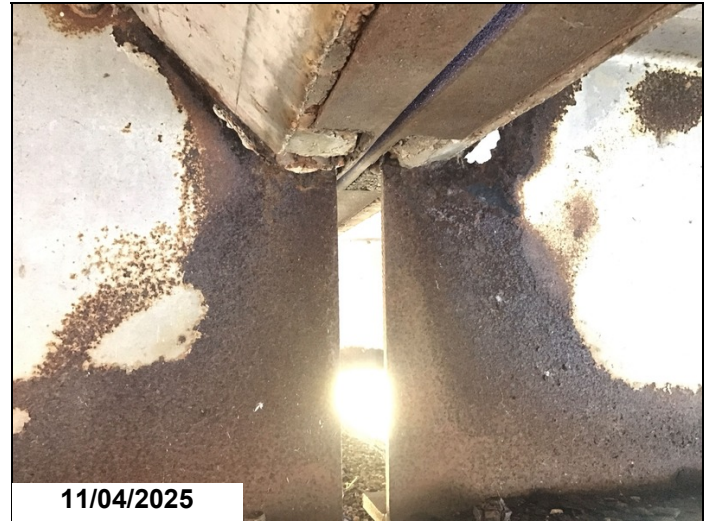
Span 10 bent 10 girder 2 has a 3" x 2" hole in web below haunch 1LF CS3.
