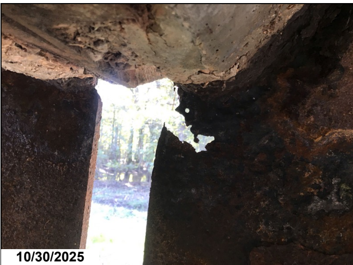
Span 16 bent 17 girder 4 has a 3" x 2" hole in web below haunch 1LF CS3.
