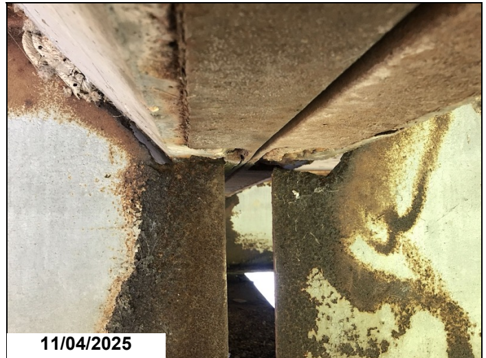
Span 21 bent 21 girder 3 has a 7" x 1" hole in web below haunch 1LF CS3.
