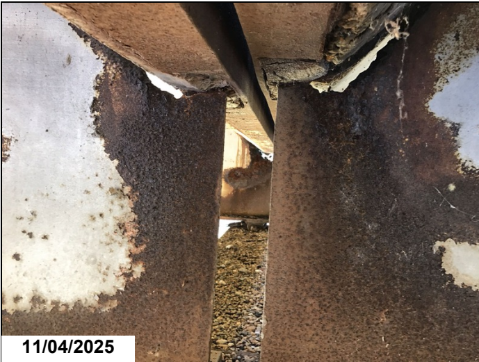
Span 18 bent 18 girder 3 has a 7" x 1" hole in web below haunch, with a 3" crack running back 1LF CS3.
