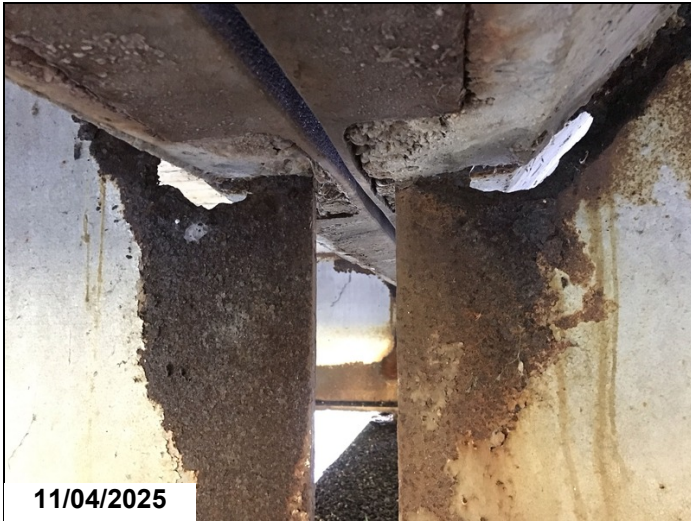
Span 11 bent 11 girder 3 has a 9" x 1" hole in web below haunch, with a 2.5" crack running ahead 1LF CS3.
