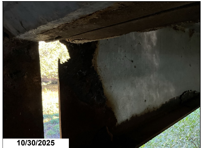
Span 11 bent 11 girder 1 has a 3" x 4" hole in web below haunch 1LF CS3.
