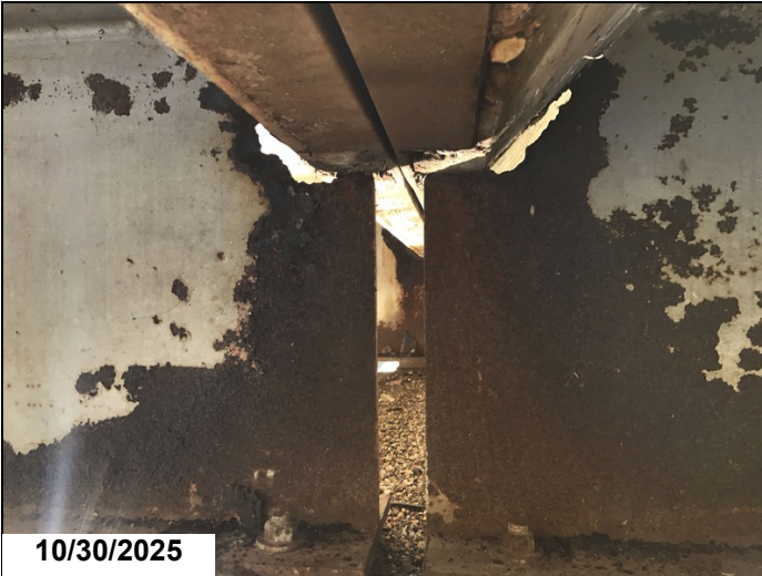
10/30/2025 Span 19 bent 20 girder 3 has a 7" x 1" hole in web below haunch 1LF CS3.
