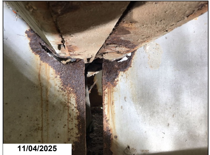
Span 20 bent 20 girder 2 has a 4" x 1" hole in web below haunch 1LF CS3.
