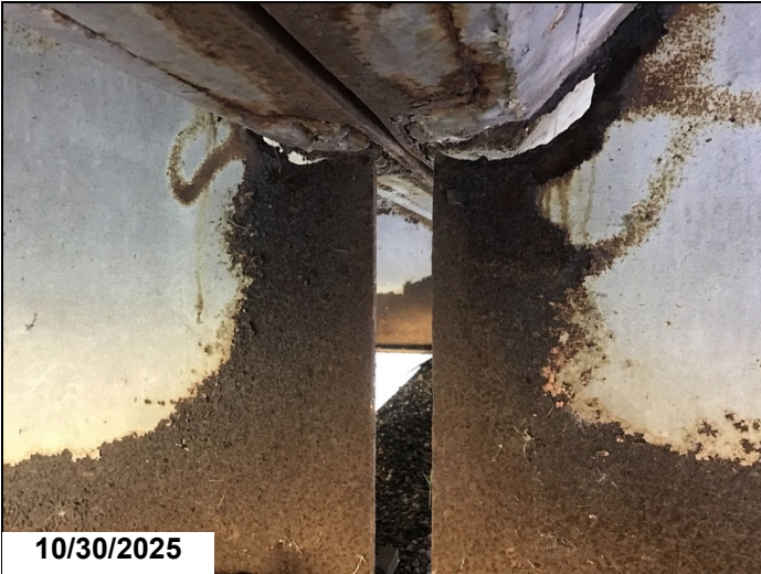
Span 8 bent 9 girder 3 has a 8" x 1" hole in web below haunch 1LF CS3.
