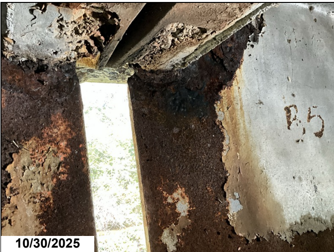
Span 12 Bent 12 Girder 1 1" diameter hole in web below haunch.
