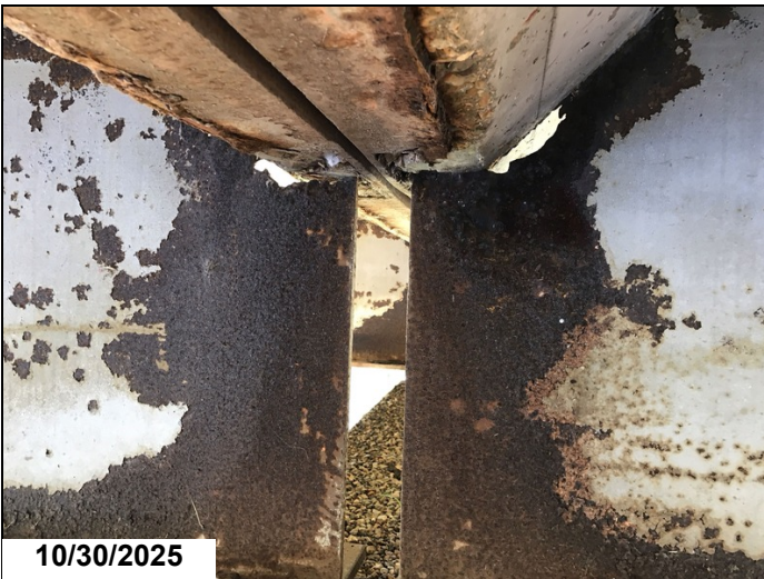
10/30/2025 Span 18 bent 19 girder 3 has a 4" x 1" hole in web below haunch 1LF CS3.
