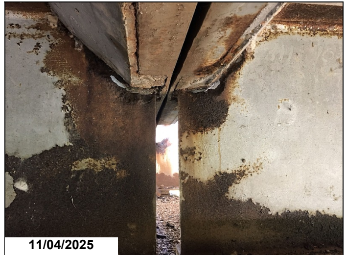
Span 16 bent 16 girder 2 has a 5" x 1in hole in web below haunch, with a 2" crack running ahead 1LF CS3.
