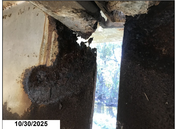
Span 18 bent 18 girder 4 has a 6" x 3" hole in web below haunch 1LF CS3.
